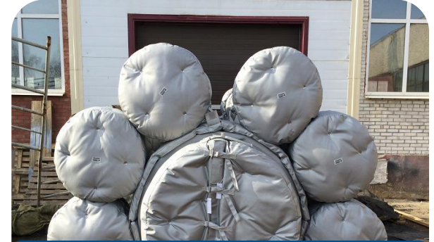
National gas company stabilizer thermal insulation
