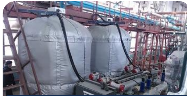
Leading Russian chemical company receiver thermo insolation
