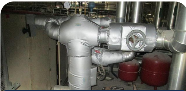
Candy producer cold armature thermo insolation
