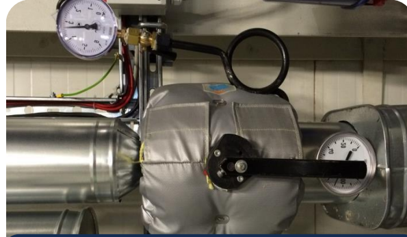
Leading German auto producer steampipe thermo insolation
