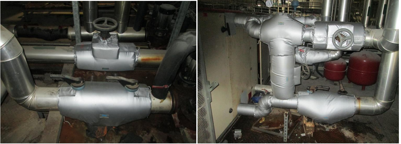
9. Manufacturer of confectionery products. Thermal insulation of cold fittings.
