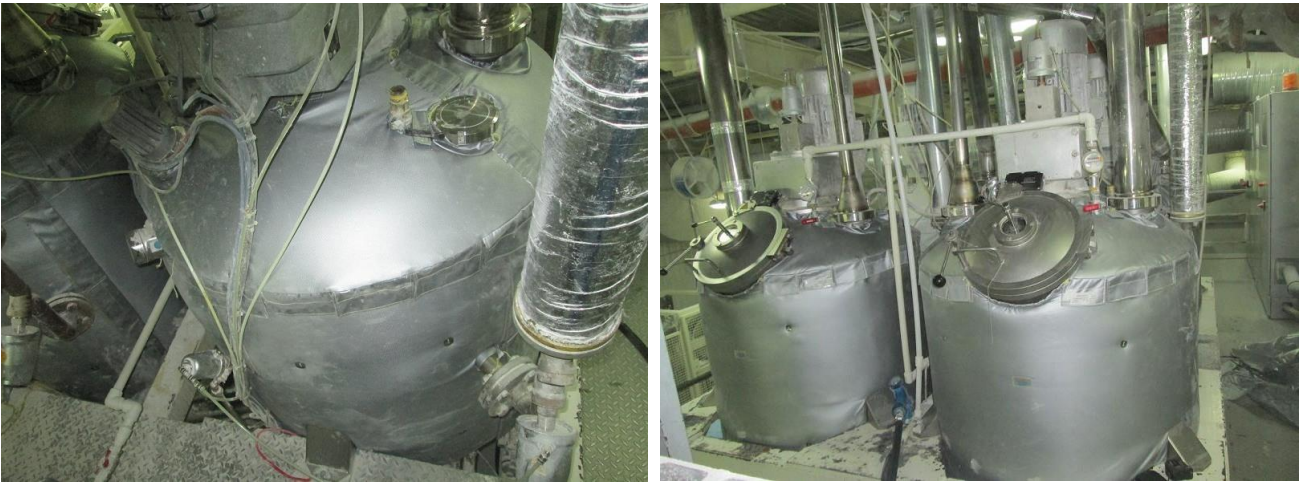
15. Manufacturer of confectionery products. Thermal insulation of boilers.
