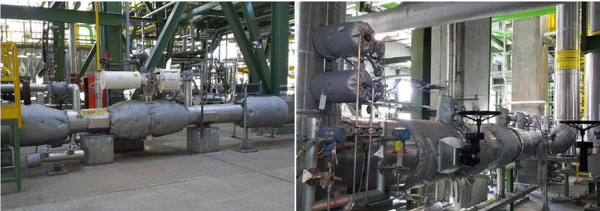
19. Chemical company in Tolyatti. Thermal insulation of fittings on hot pipelines.
