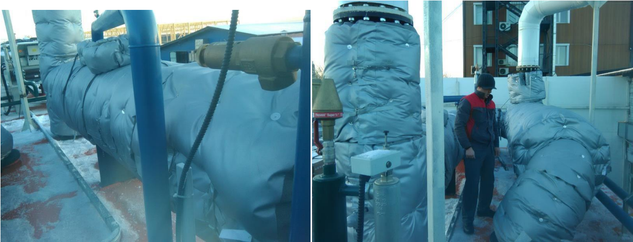
6. Engineering company. Thermal insulation of the exhaust system.
