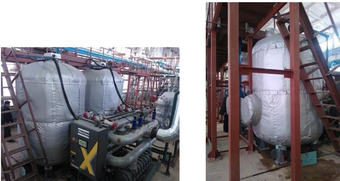
17. Leading Russian chemical company. Thermal insulation of receivers.
