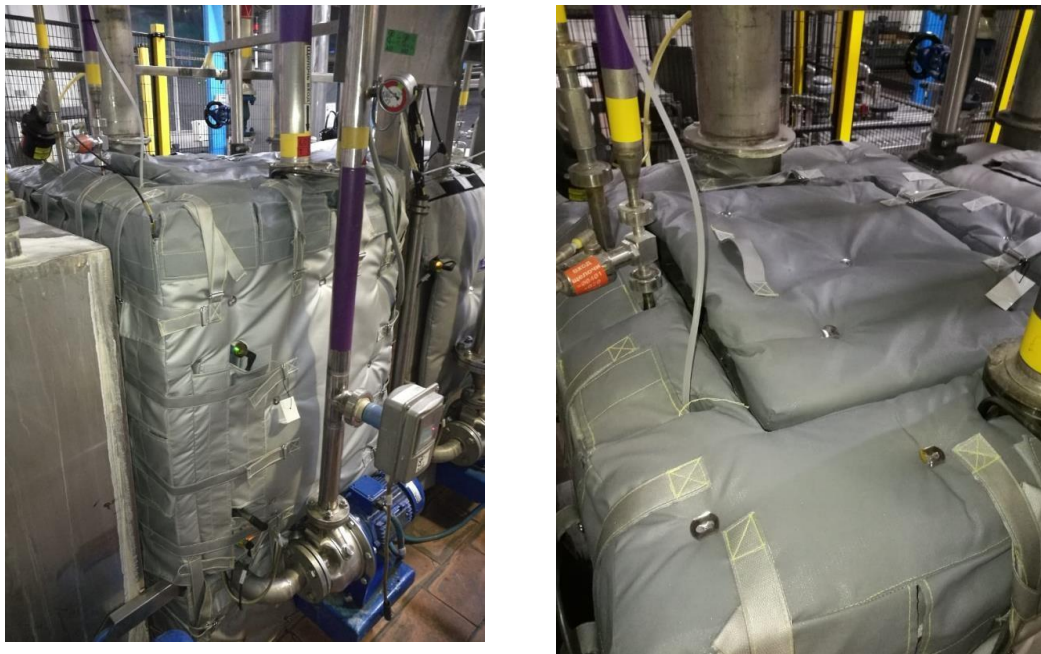
21. Food company in the Sverdlovsk region. Thermal insulation of alkaline process tank.
